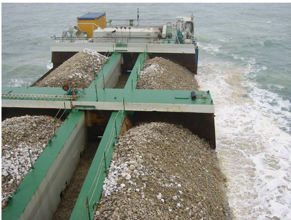
Figure 4 Dumping of filter stones. The stones are 30 – 200 mm with an average ( d_{50} ) of 100 mm.
