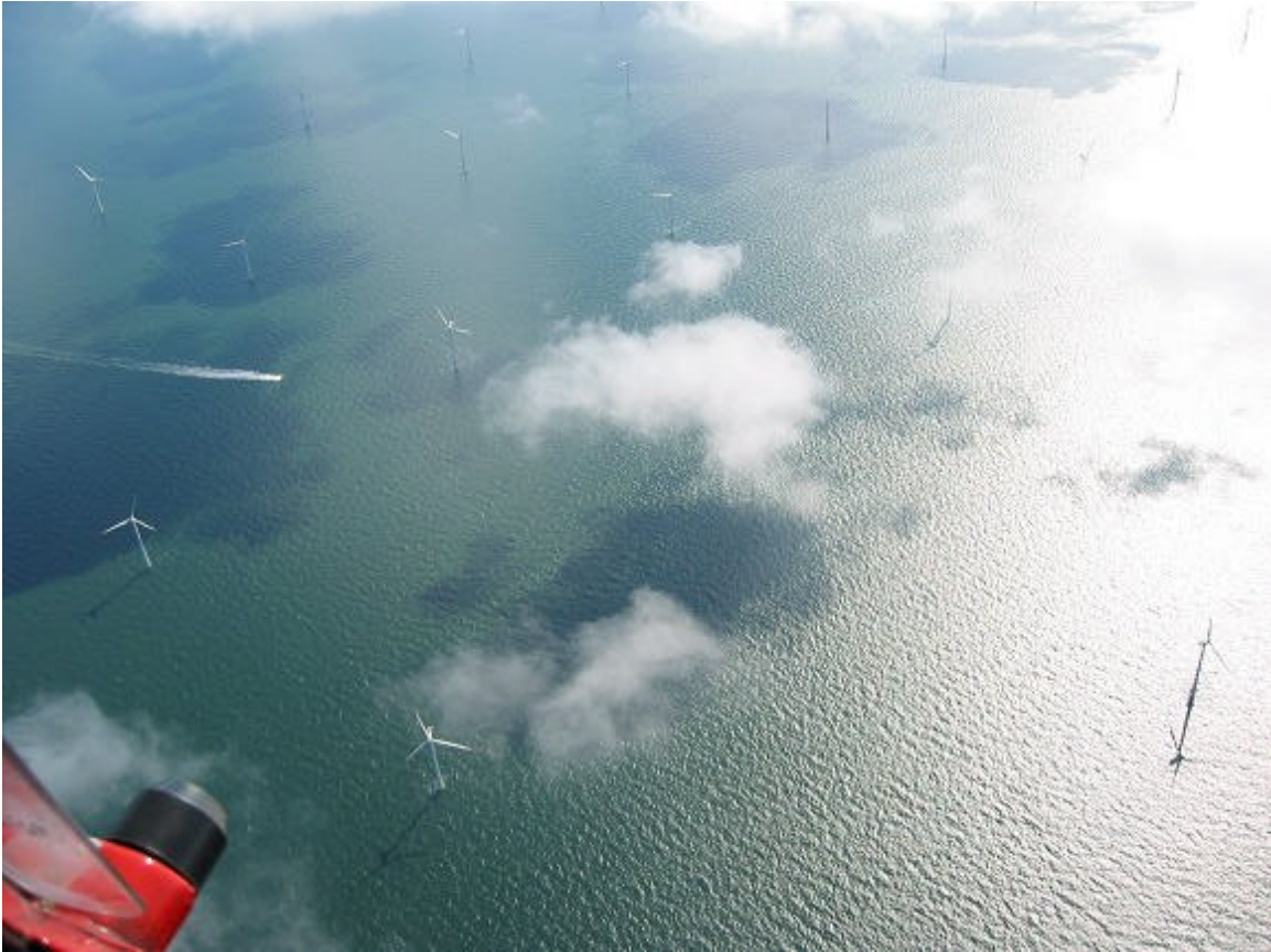
Figure 13 Seen from above it is clear that the turbines do not cram the ocean.
