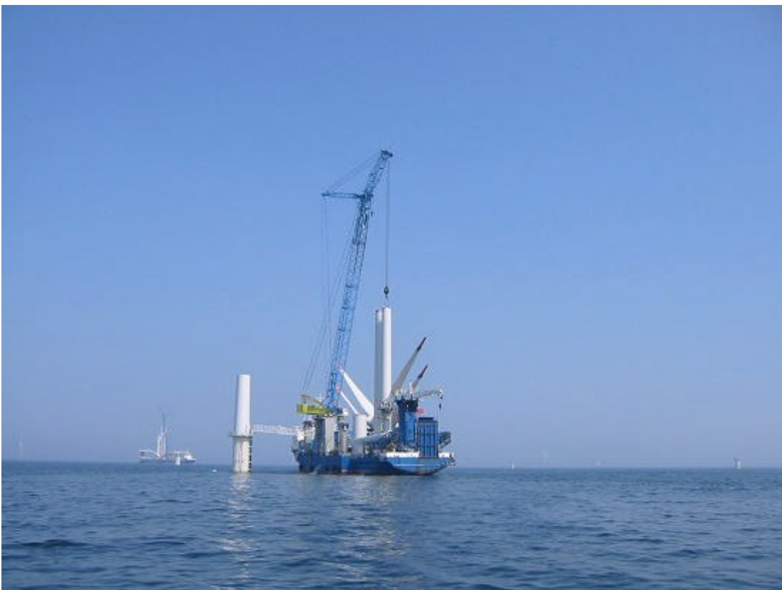
Figure 10 Turbines were transported to the site and erected by 2 purpose-built ships.
